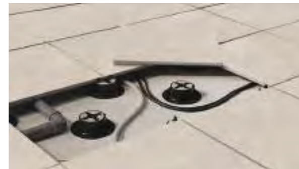
Laying as raised paving. Colocación sobreelevado.
