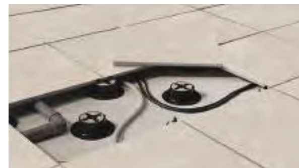
Laying as raised paving. Colocación sobreelevado.
